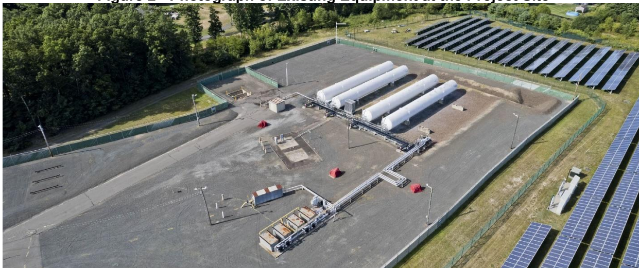
Figure 2 - Photograph of Existing Equipment at the Project Site
