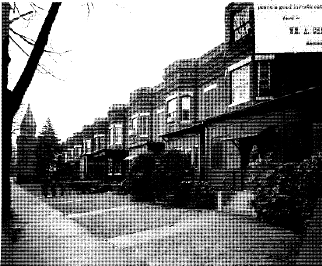
1986 - Same cottages as shown above are still in use on Walnut Street in Holyoke
